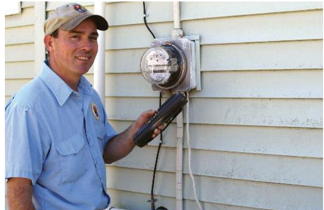
A Meter Reader inputs the electric meter data from this home. When he finishes his daily route, he can place the Itron data unit into a docking station and automatically download the current data.
