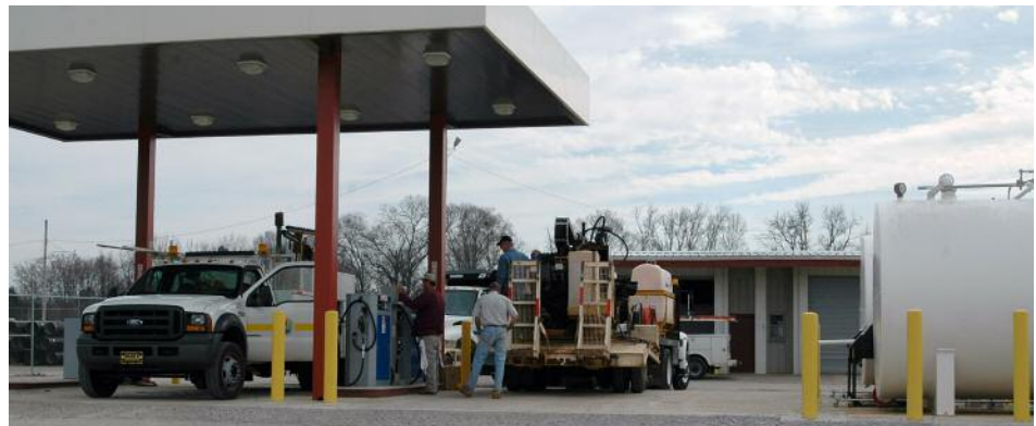
The Natural Gas Department financed the installation of a fuel station at the water and gas facility. This helps ensure availability in times of crisis as well as helping control the cost of fuel.
